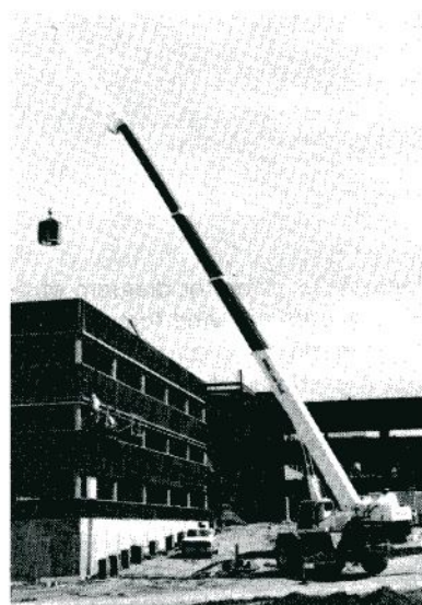
Figure 4-1. This telescoping boom crane can lift weights of more than 17 000 newtons to a height of sixteen stories.
